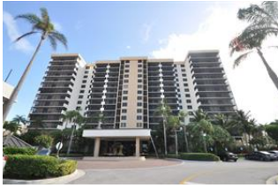
Front of Building
