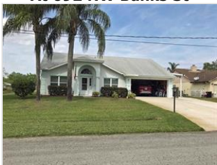
Neighboring Homes On NW Banks St.
